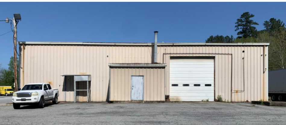
Rear Service Building
