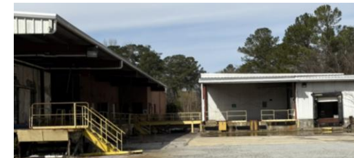
Rear of Building B
