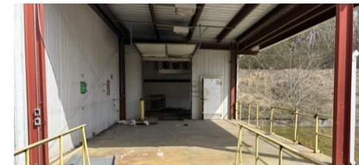
Loading Area of Building B
