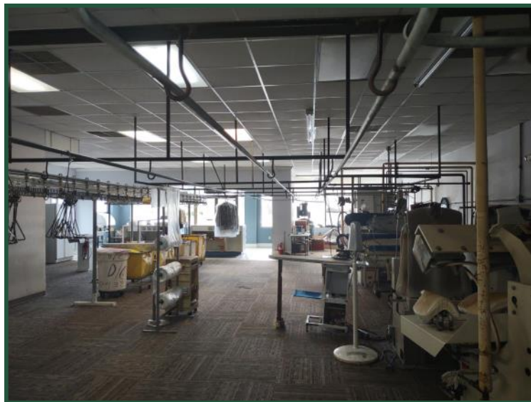
Interior - From Rear
